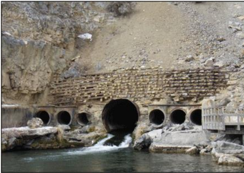
Photo 3b (3/27/2013) – Similar view of the tunnel outfall at low flow conditions.
