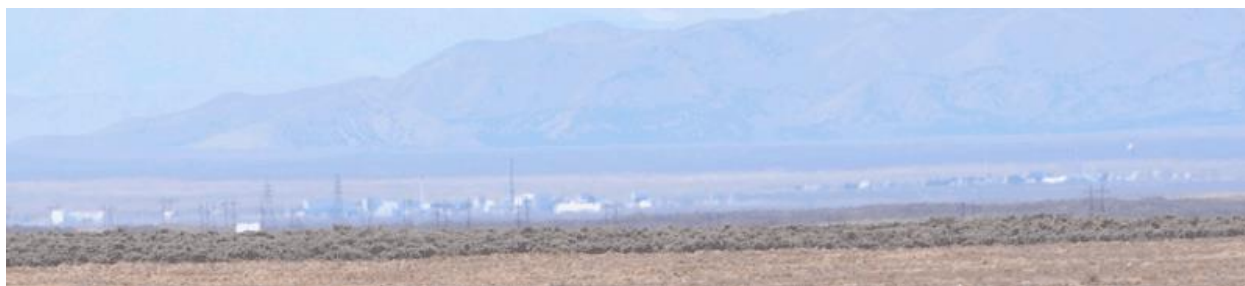
Idaho National Laboratory INTEC and ATR Complex.
